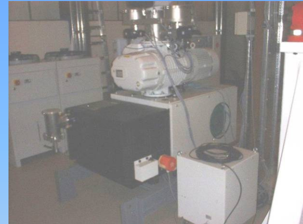
Roughing Pumps (Leybold)
