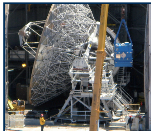
SCUBA-2 being lifted into the JCMT enclosure (3rd April 2008)
